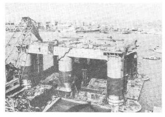
The Kantan No. 3 semi-submersible oil rig, China's first, constructed by the Shanghai Shipbuilding Plant. Xinhua
