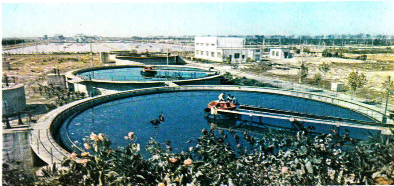
Sedimentation tanks in the waste water treatment plant.
