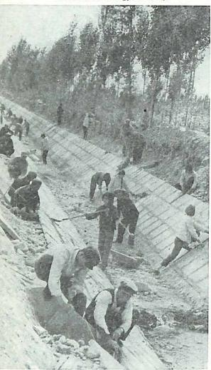
channels were reconstructed into 13 new trunk canals. The large Yingko Canal built during the Tang dynasty had fallen into a deplorable state, its dyke crumbling at many places. It was practically dry in the summer. Autumn floods breached the dyke and submerged villages and large tracts of land. Dredging and reconstruction done during the cultural revolution doubled its diversion capacity so that 4,700 hectares of land belonging to four communes were brought under irrigation.
