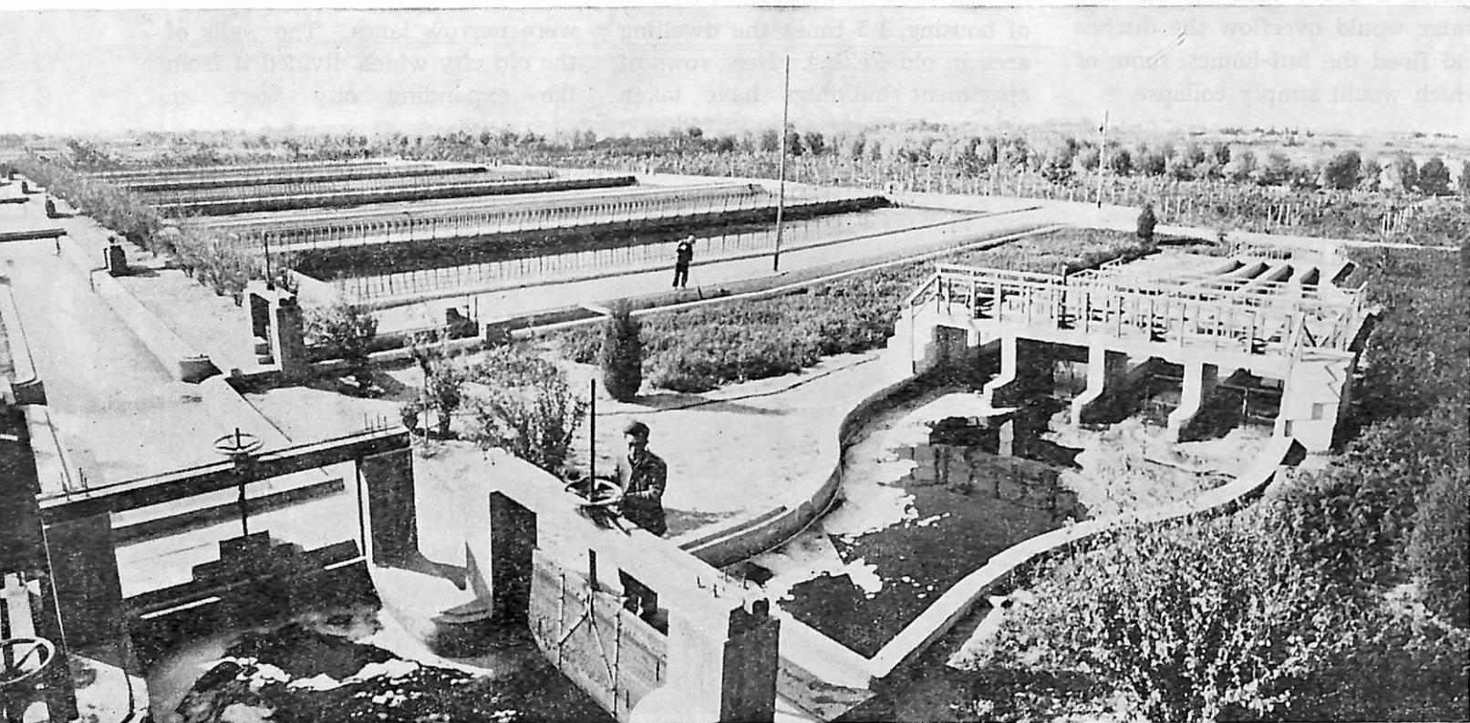
A station for treating the city's waste water built in the suburbs.
