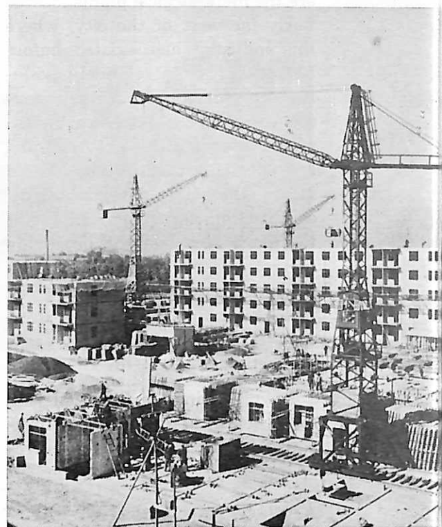
Apartment blocks being built on the eastern outskirts of the city.
