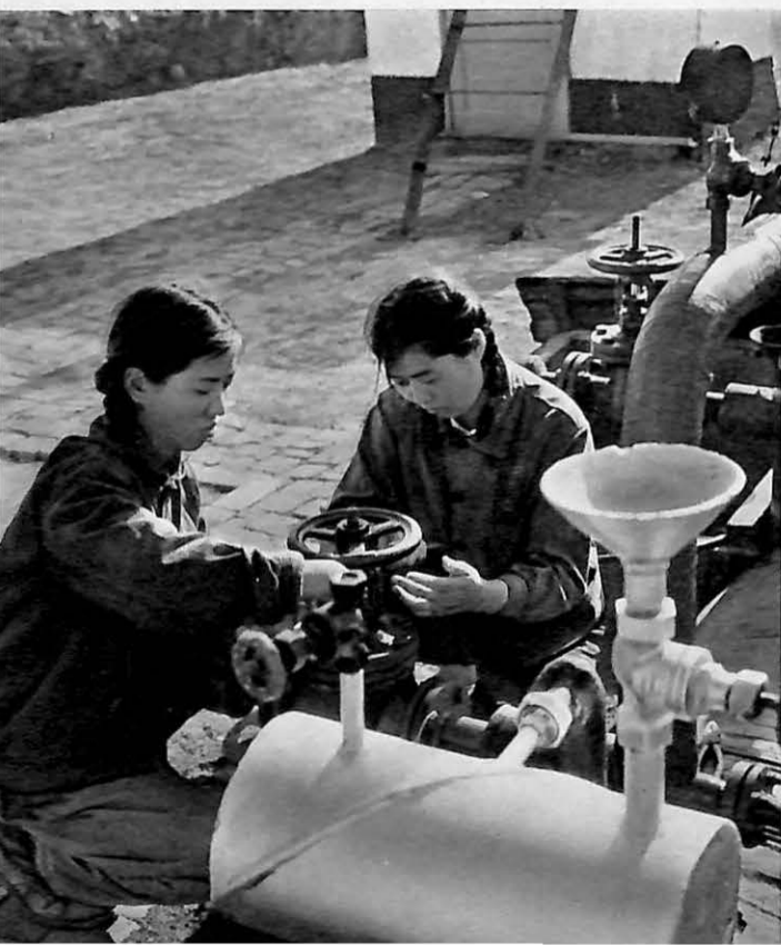
Checking and repairing an oil-well installation.
