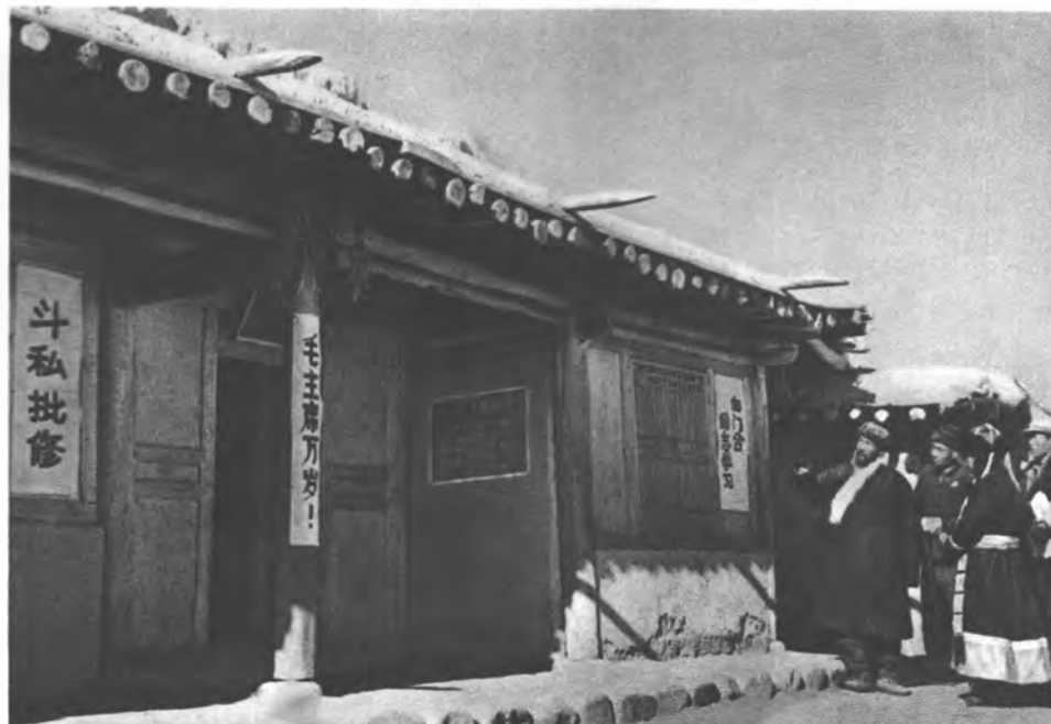
The new houses Comrade Men Ho mobilized the brigade members to build for two old poor peasant families.
