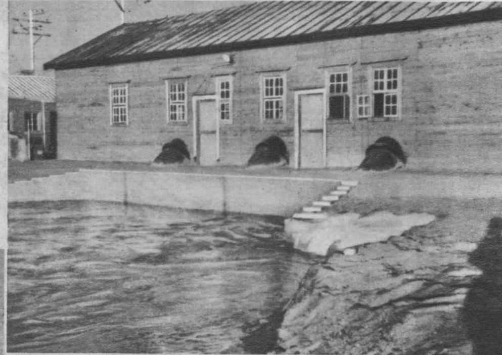
The pump house of the Taku salt fields. During high tide the sea rises, flows into a canal and is then pumped into the reservoir
