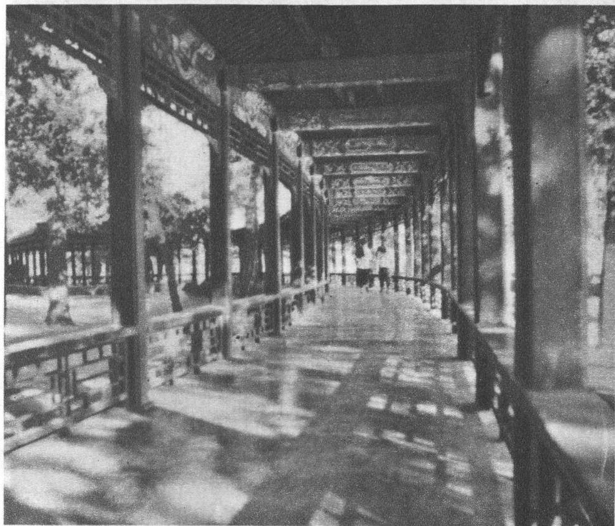
The long Veranda skirts the lake by the foot of Wanshoushan. It is more than 1440 feet long, with a brilliantly painted ceiling
