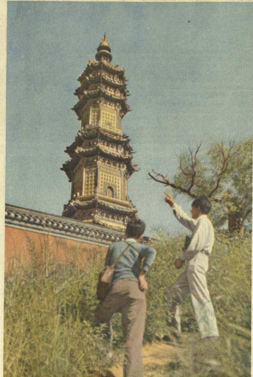
The To Pao Pagoda is faced with yellow glazed-tiles, surmounted with a golden crown and is 120 feet high
