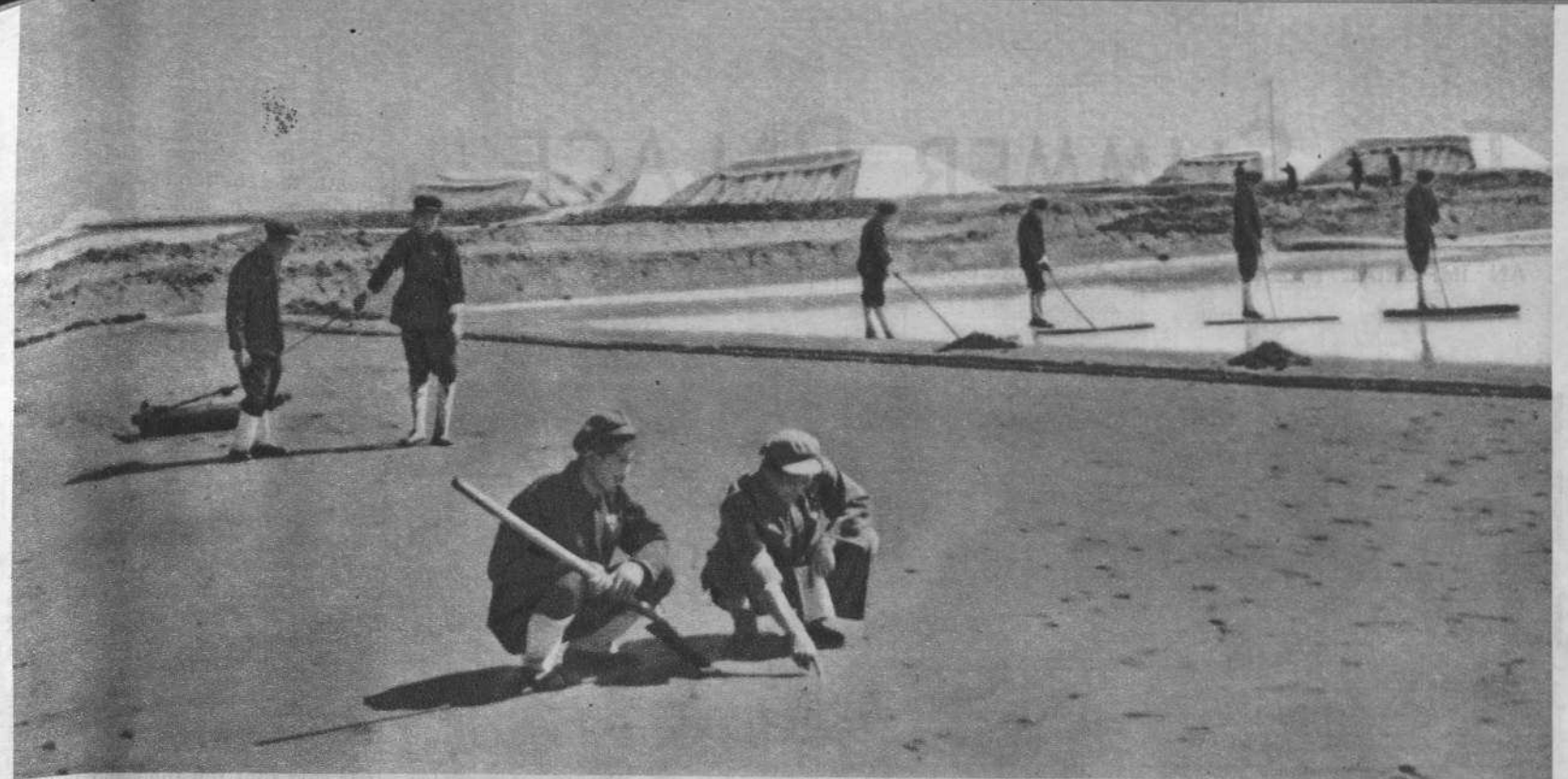
Careful preparation of the pond-bed is important for rapid crystallisation. Departmental head Tang Chung-yao (right) and technician Tung Shou-lan (left) inspect the bed to see if it is up to standard
