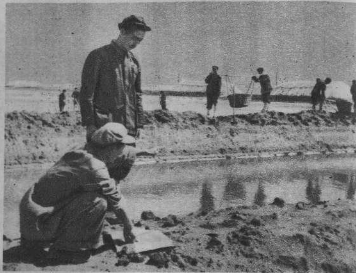
Preparations for enlarging the brine pools for next year's increased production. Salt drying finishes in autumn; but brine is left in the pools for the production of saltpetre for industrial use
