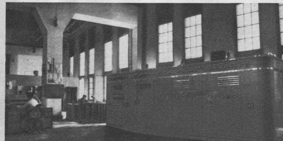
The 7.5 kilocycle shortwave transmitter of Radio Peking, built by the People's Radio Factory. Shortwave transmitters carry sound for thousands of miles in wireless waves in a series of ricochets between earth and sky
