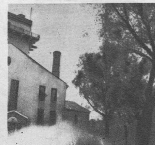
A newly-built fountain at Radio Peking is used to cool the transmitter
