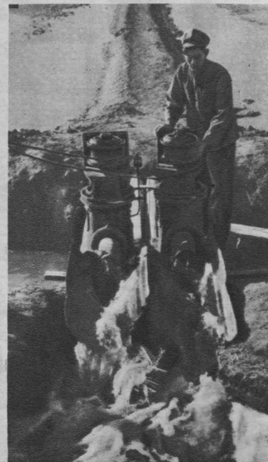
One of the newly installed electric pumps on the Taku salt fields
