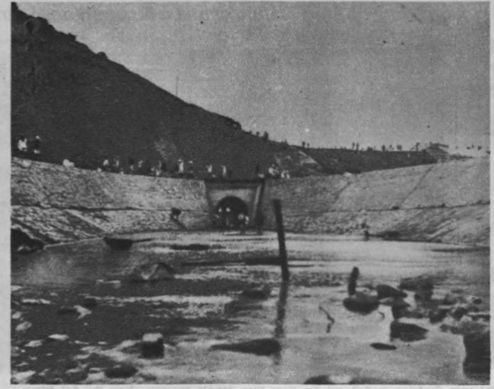
The outer end of the Shihmantan water-tunnel in construction
