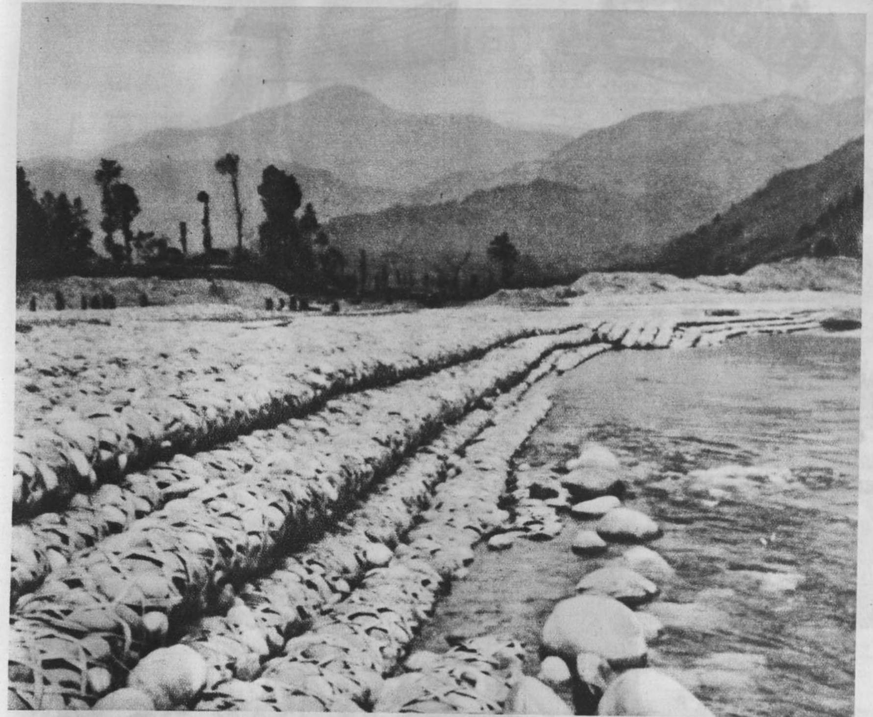
Felsayen Dam spills the overflow from the Inner Canal to the Outer, acts as a flood control
