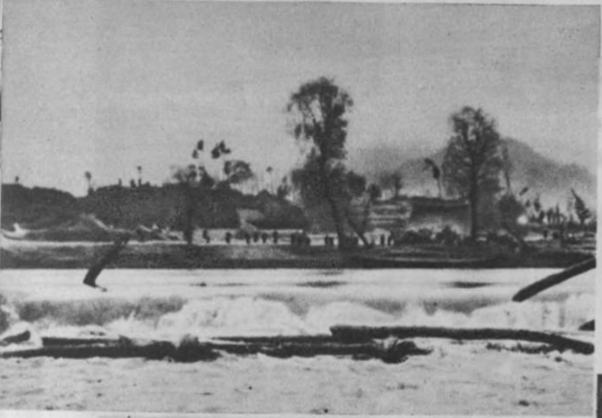
The 'Matza' is a bamboo, earth and pebble construction which diverts the flow from one canal to another while annual repair operations are in progress. When repairs are finished the 'Matza' is removed
