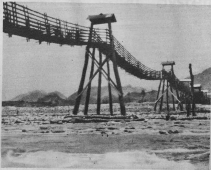
This ancient bamboo and rope bridge is still the main communication route across the Min River
