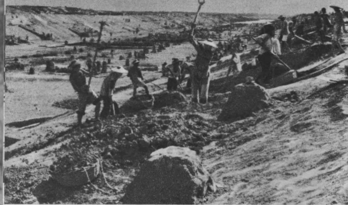
Large-scale dredging carried out by more than 200,000 peasants along the Sui River has removed the danger caused by a Kuomintang crime. When the Kuomintang breached the Yellow River dikes in 1938 its waters flooded over the plains and silted up the Sui River, one of the main tributaries of the Huai
