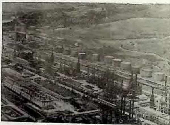
The oil-processing plant at Ballsh
